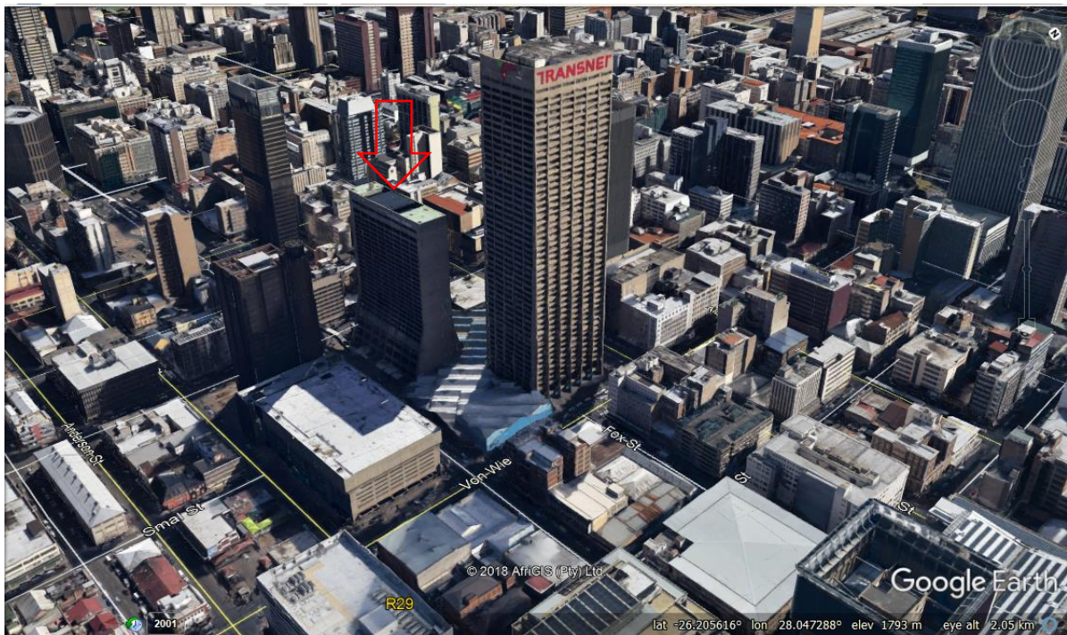
Figure 1: Carlton Hotel and Transnet (Carlton) building.
