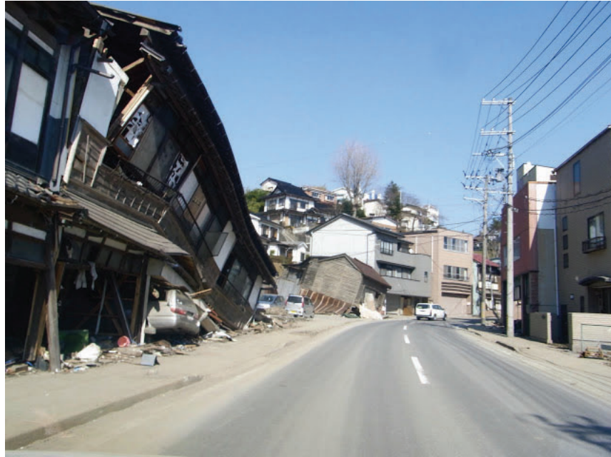
Tohoku earthquake damage
